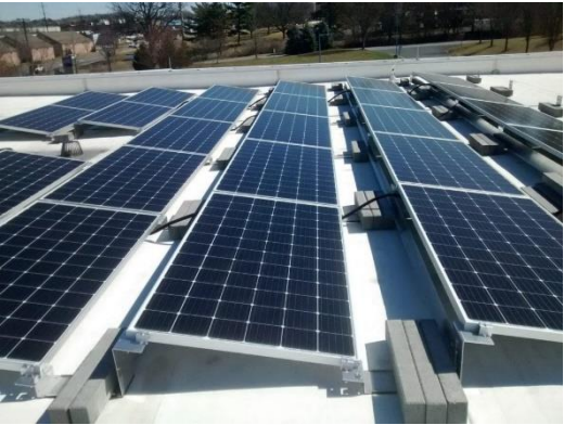
Ballasted mounting system
