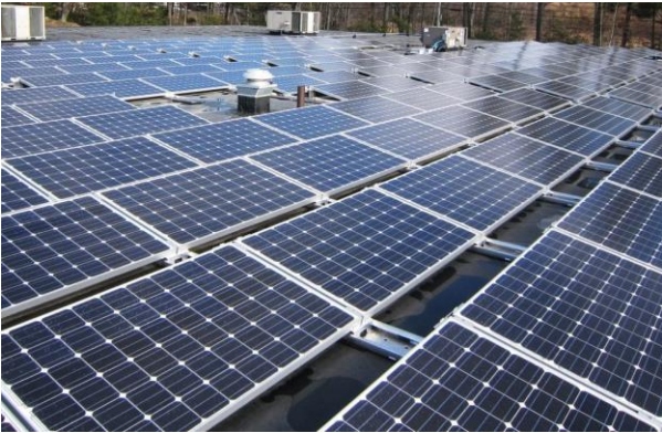
Rail-based mounting system
