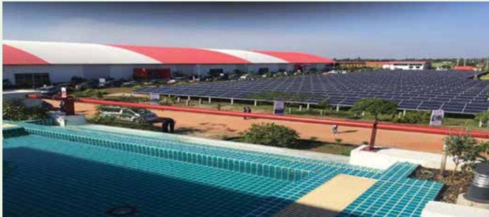
Solar Net Metering at Madhabpur, Habiganj
